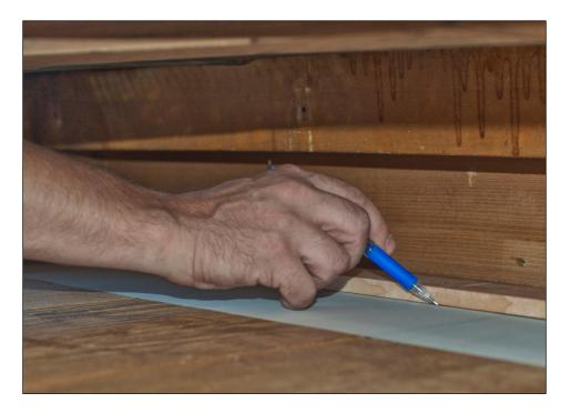
Use a straight edge and a Mylar pencil to draw a line between the note #1 and note #88 strike points on the Mylar.
